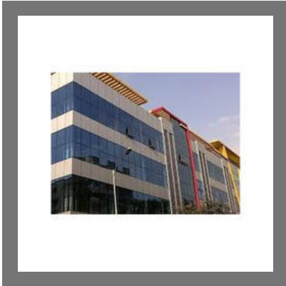
ACP Structure Glazing
